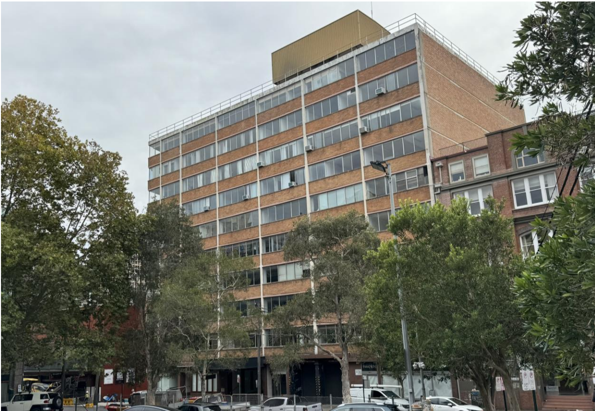
Figure 2. Looking towards the Kippax Street frontage of the site
